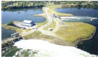
Figure 3.8 A tidal generating station transforms kinetic energy from tides to electrical energy.
